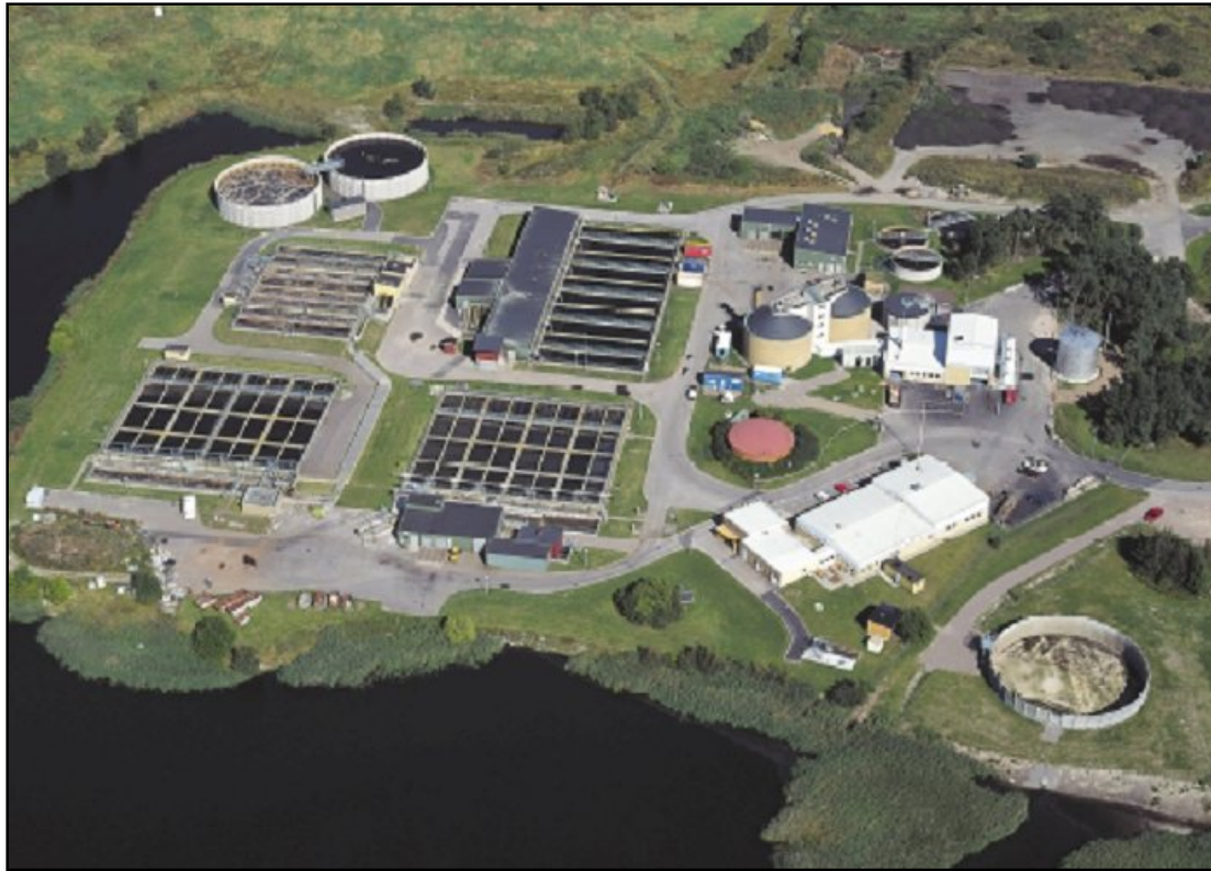
Kalmar Biogas Plant
